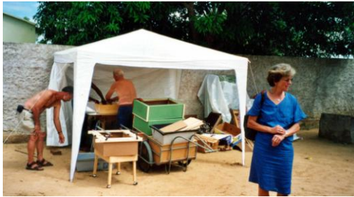
Beginning of solar cooker fabrication under a tent, in the front the initiator Regula Ochsner
