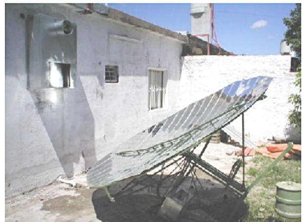
**Fig. 2. Scheffler-reflector and cooking place jutting out of the wall**
