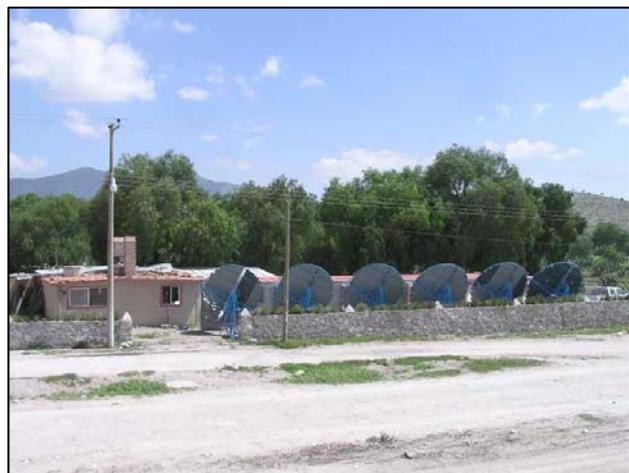
After some no satisfying attempts to process the syrup with small solar stoves (SK-14) in 1999, new efforts in 2005 with Schefflerreflectors were successful. In 2008 started the production of solar agave syrup with six 10m<sup>2</sup> Schefflerreflectors in a new kitchen building.
