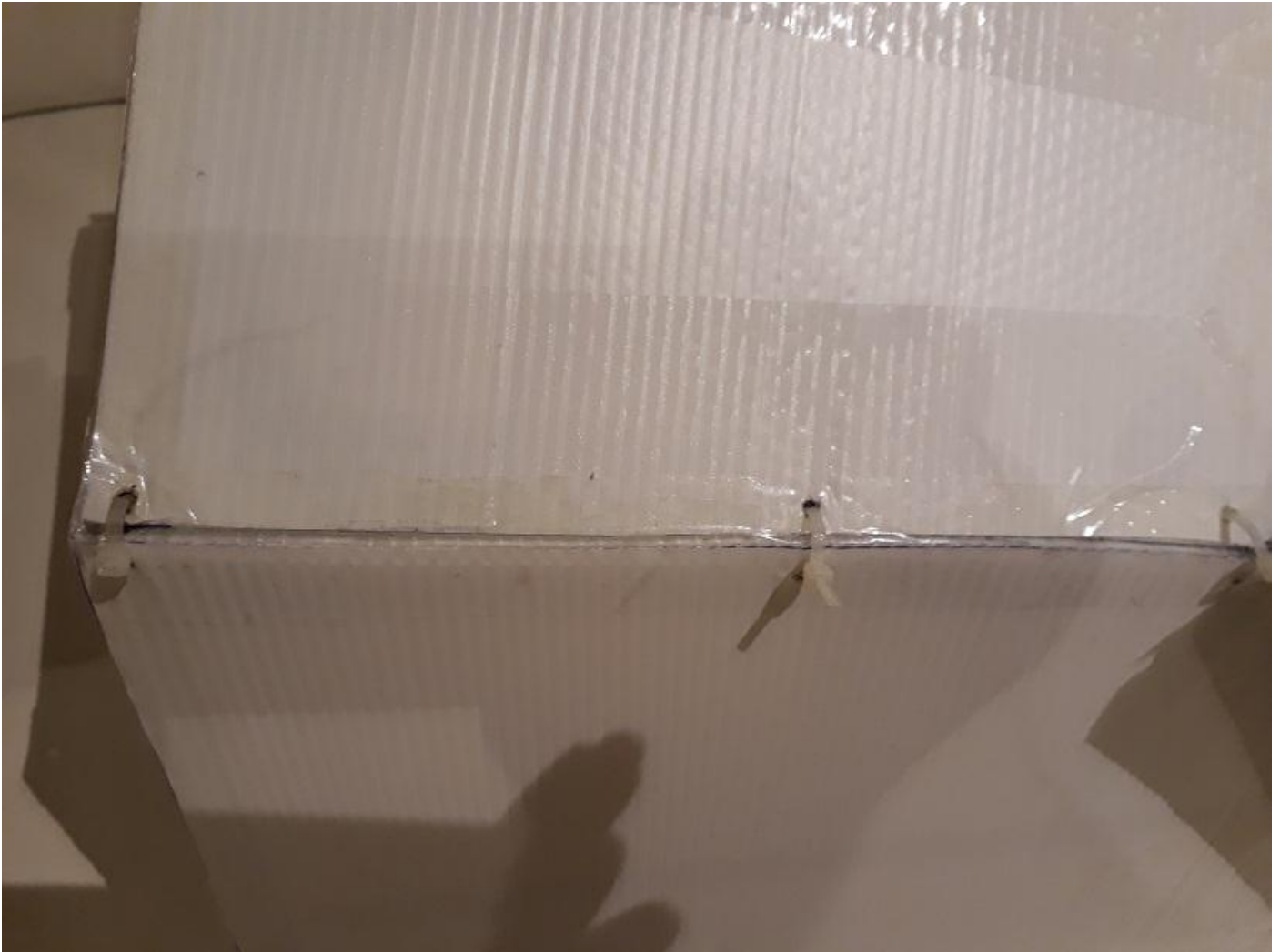
Fig 11 – Detail of using zip ties to join petals or sides of SC. Zip “heads” stay outside
