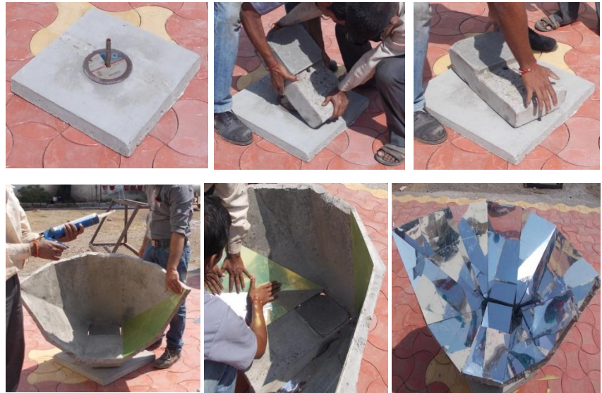
Simple construction, appropriate technology
