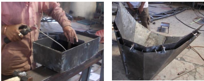
Moulds manufactured using appropriate technology
