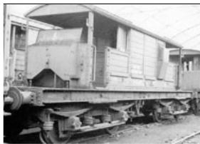
Built in 1936, this Southern Railway bogie goods brake van was rated at 25 tons. The van section is of 'normal' length with exceptionally long verandahs to put the guard's door over the bogie centres. Not the large sand hoppers on the exterior of the verandah. This example was photographed as late as 1964.
